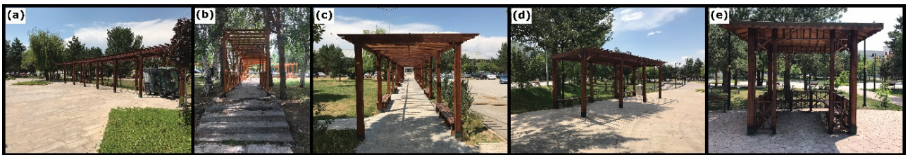
Figure 8. Top Cover Elements in Atatürk University Building
