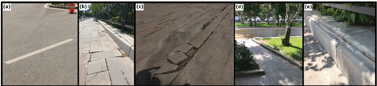
Figure 2. Vehicle Road-Asphalt (a), Pedestrian Crossing-Concrete Slab (b,d), Pavement-Concrete Slab (c), and Curb-Concrete (e)
