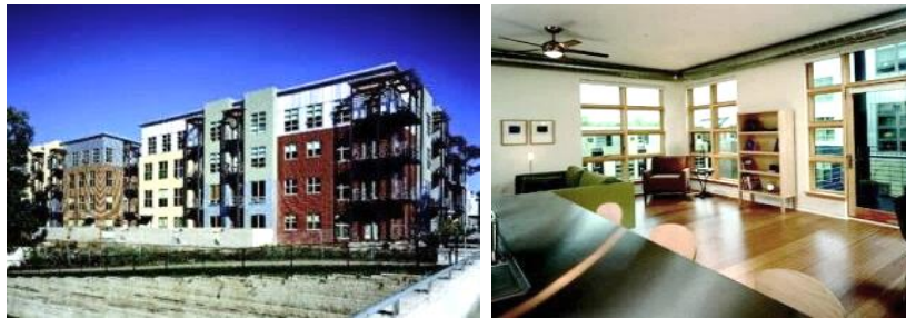
Figure 1. ERD Building; MIDTOWN LOFTS, Minneapolis (Url-1)
