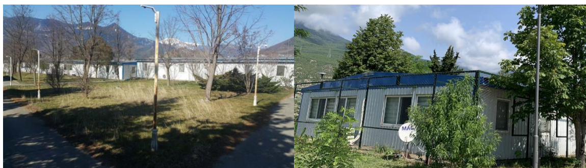
Figure 5. Administrative - Education and Research Buildings
