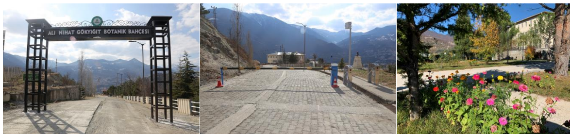
Figure 4. General view of the entrance gate and its surroundings
