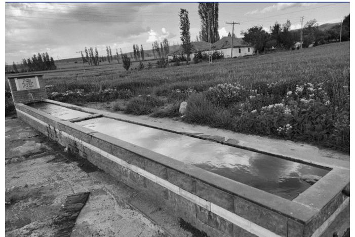
Figure 2. Two-partition concrete water trough.
