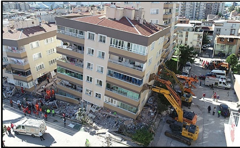
Şekil 12: Deprem sonucu aldığı hasar (BBC News Türkçe 2020) Figure 12: Damage as a result of the earthquake (BBC News Turkish 2020)
