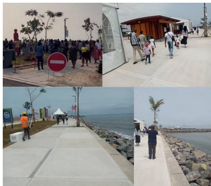
Figure 14. The northern promenade. The pictures were taken on 20 August 2022, during the opening ceremony.
