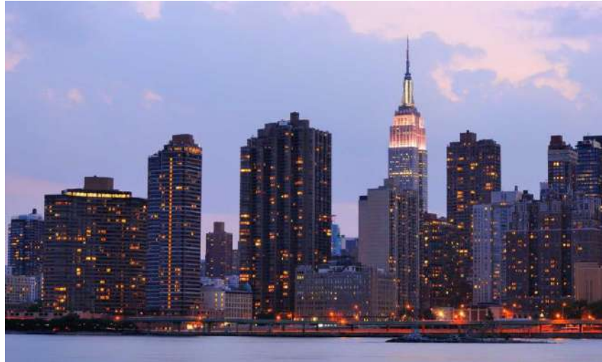
Figure 2. Empire State Building, New York [6]
