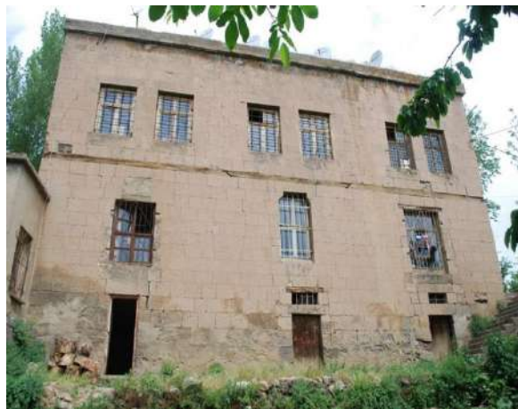
Figure 5. Zeydan neighbourhood, block 499 parcel 7, double window row on the 1 st floor façade (source: author, 2013)
