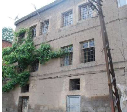
Figure 4. Zeydan neighbourhood, block 456 parcel 1, double & triple windows on the façade (source: author, 2013)
