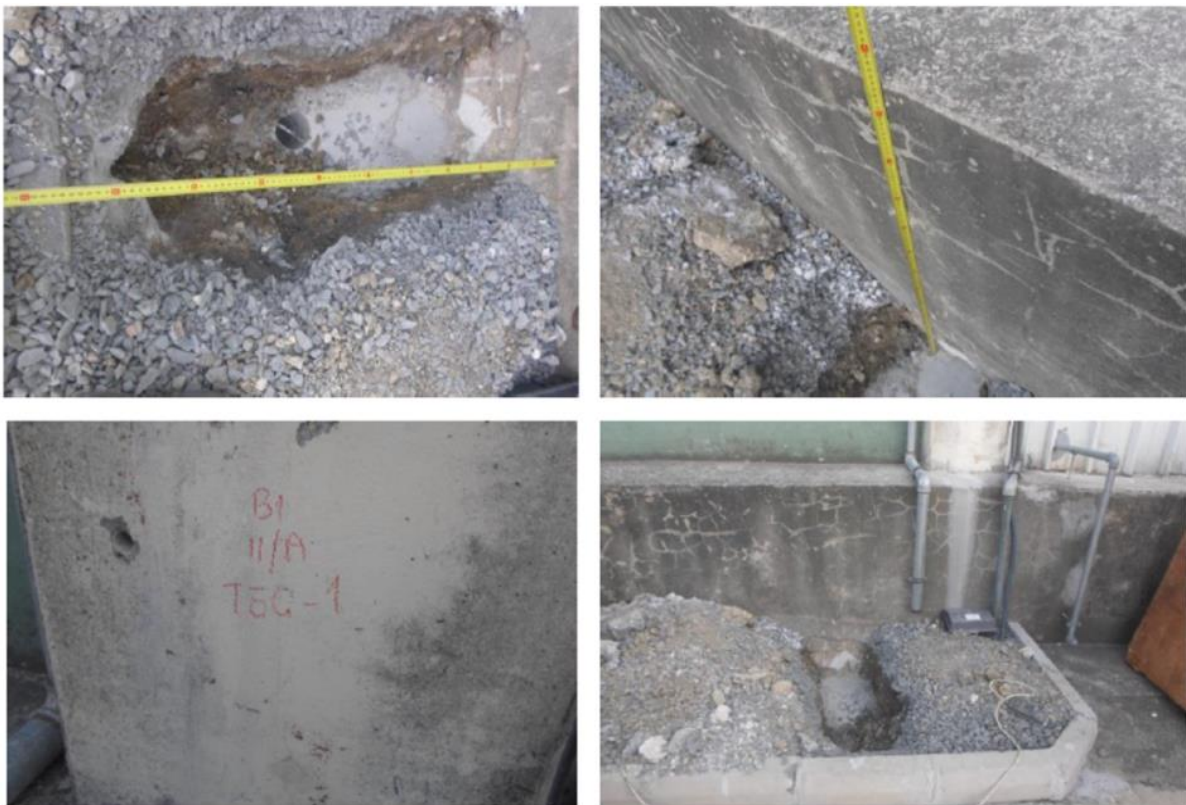
Figure 3. Foundation test pit excavation
