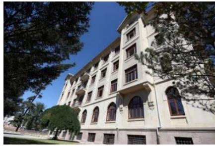
Figure 18. On the front facade of Ankara Medipol University Rectorate Building [25].
