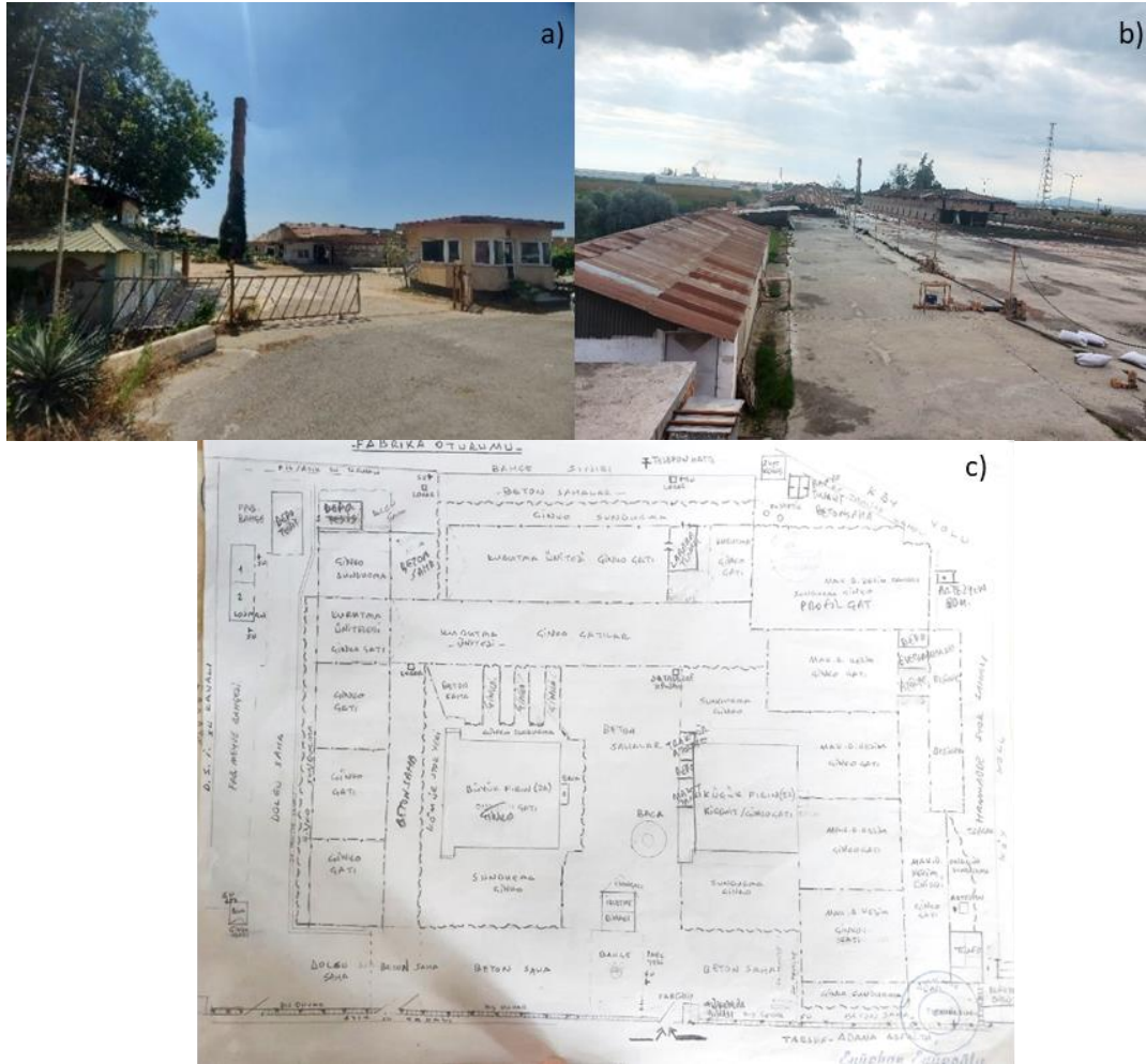
Figure 3. a, b) General Views of the Factory Campus; c) Unscaled Sketch of the Factory (Eyüpoğlu E.)
