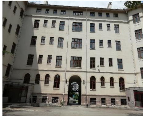
Figure 21. The inner courtyard facades of Ankara Medipol University Rectorate Building [28].
