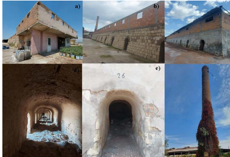
Figure 7. a) Small Kiln Appearance; b,c) Large Kiln Views; d,e) Kiln Chamber Views; f) Chimney Drying Areas: After the kilns, the most unique building unit of the campus is the drying area. The drying process is carried out in semi-open areas with a concrete floor, built on reinforced concrete columns and beams, with wooden roof trusses, covered with metal sheets (Figure 8a,b,c,e,f).
