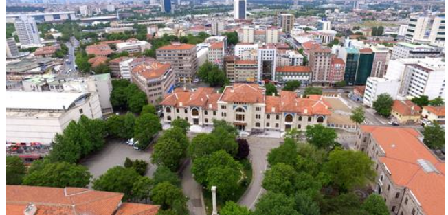
Figure 24. General view of the area where Ankara Social Sciences University Rectorate Building is located within the city [30].
