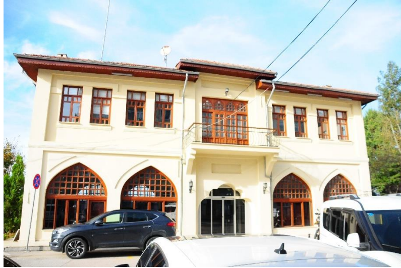
Figure 14. Rear Facade - Southeast Facade
