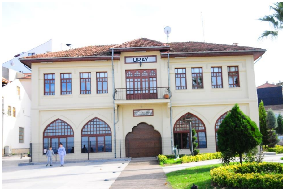
Figure 13. Entrance Facade - Northwest Façade
