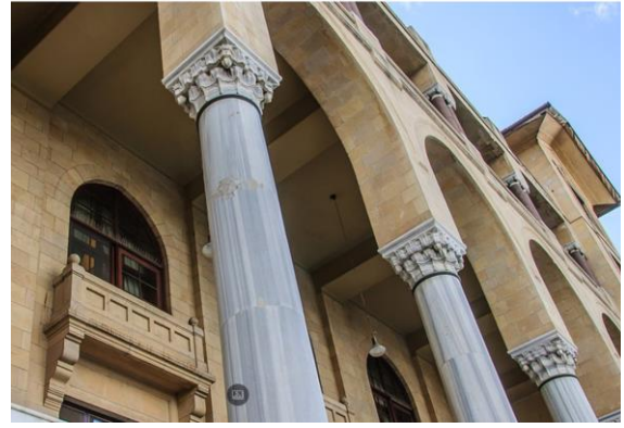
Figure 6. Marble Column Detail in Gazi University Rectorate Building [18].
