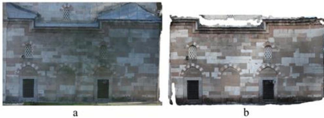
Figure 7. Orthophotos of the west façade. a. produced from UAV and b. produced from TF.
