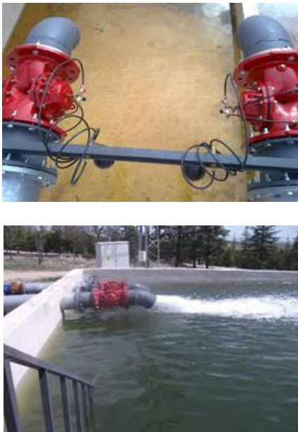
Figure 10. Float valves
