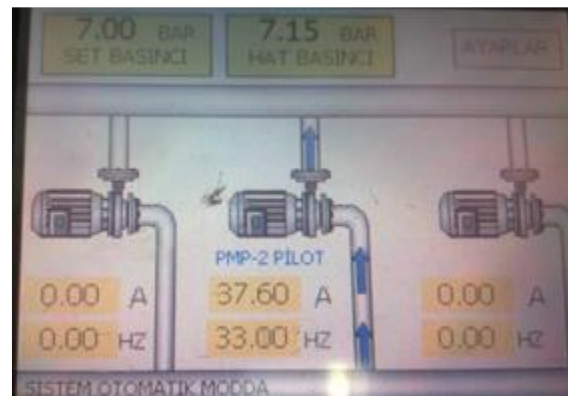
Figure 5. PLC used in an irrigation pumping plant
