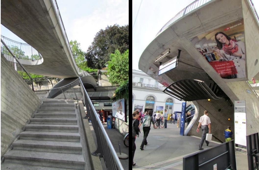
Figure 7. Stadelhofen Station, Curves (Photo taken by the author, 2013).
