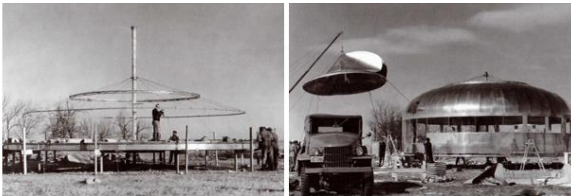
Figure 12. Construction Steps of the Dymaxion House (Altın, 2013).
