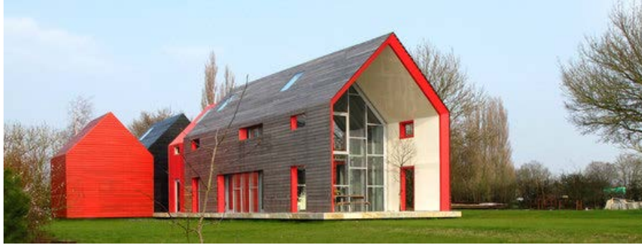
Şekil 7. dRMM Architects, Sliding House (URL-7)
