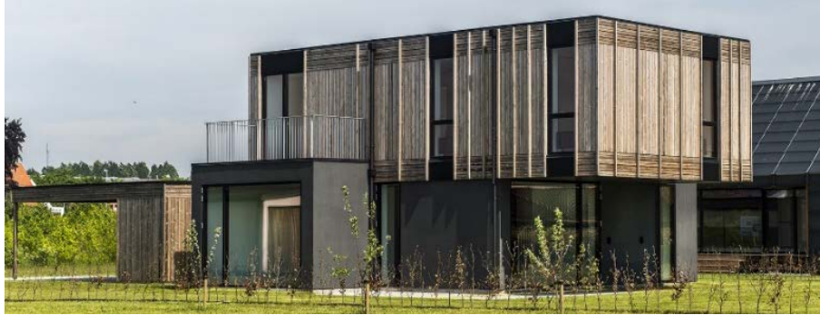
Şekil 6. Henning Larsen Architects, Nyborg Adaptable House (URL- 6)
