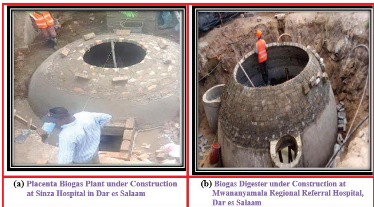
Figure 2. Biogas plants at two Tanzania hospitals [From Honest & Saria [240] & Kellner [243], with permission from JEP & GHW, respectively].
