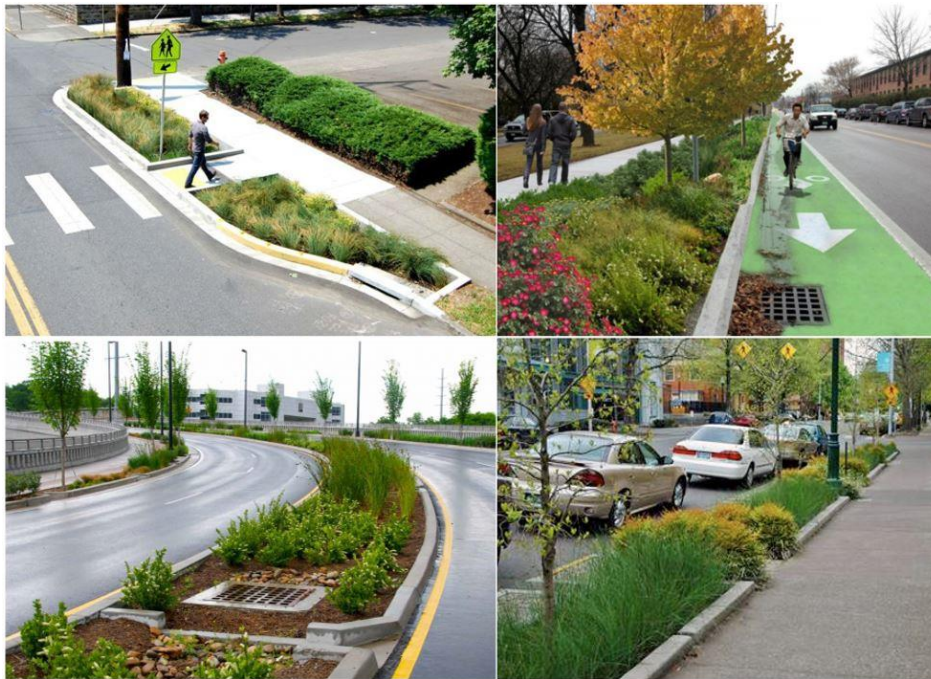
Figure 3. Examples of Green Streets from Various Locations: Curb Extension and Arterial Swales in Vermont (Top Left & Right) (URL 5) Median with Bioretention Planters in Philadelphia (Bottom Left), (url 6). Infiltrated Planters in Portland (Bottom Right), (URL 7).
