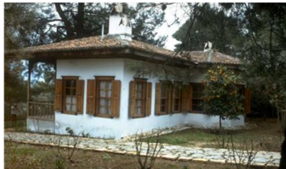
Figure 6. Side elevation showing the wooden eaves; Mugla chimney and rectangular wooden Windows (Çakırhan, 2005).
