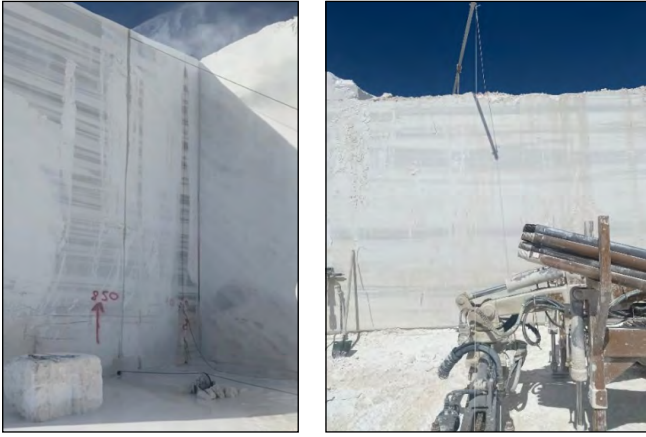
Figure 4. Vertical cutting and horizontal diamond wire cutting process
