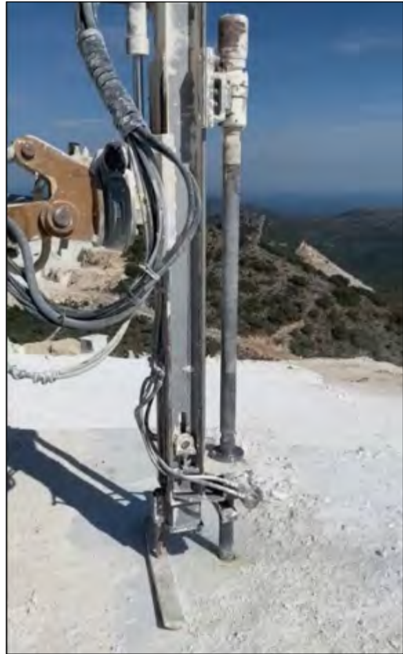
Figure 3. Image of drilling a vertical hole in a marble block
