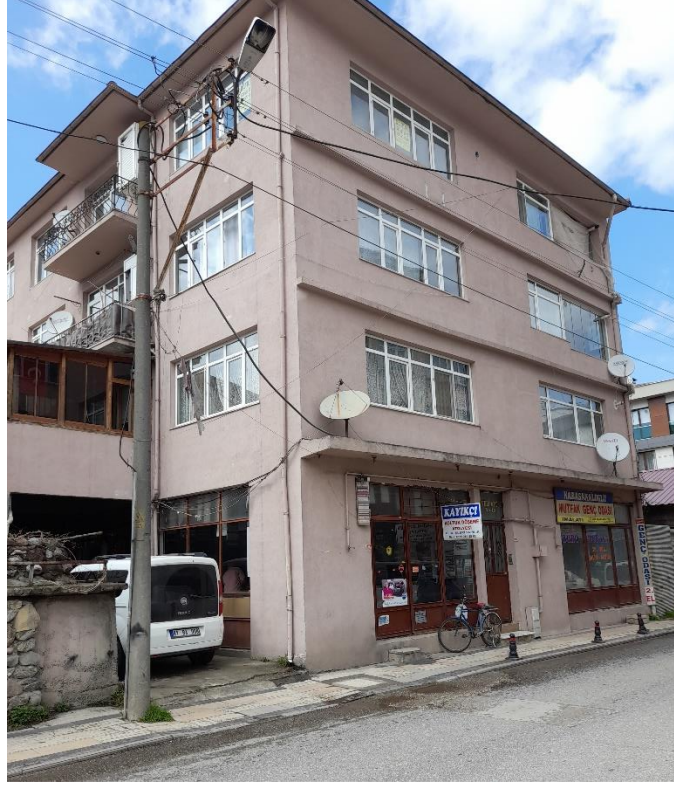
Figure 3. View of the examined building from the road front
