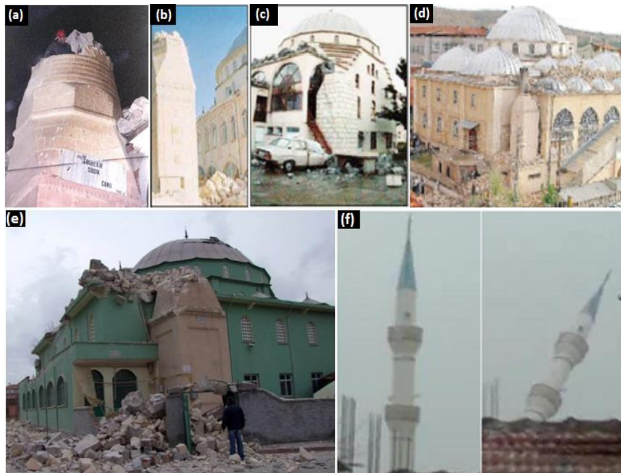
Figure 1. Minarets damaged by wind, (a) Ebubekir Sıddık Mosque/Ankara-Kayaş, (b)-(c) Mersin-Erdemli, (d) Ulu Mosque/Kahramanmaraş, (e) Kurtuluş Mosque/Kırıkkale, (f) Şafak Mosque/İzmir, (g) Ordu-Ulubey, (h) Niğde, (i) Aydın/Nazilli
