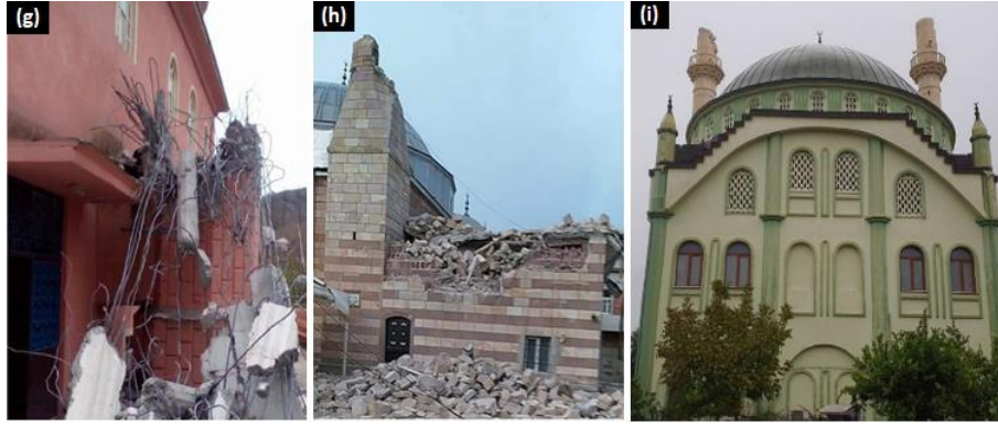
Figure 1. Minarets damaged by wind, (a) Ebubekir Sıddık Mosque/Ankara-Kayaş, (b)-(c) Mersin-Erdemli, (d) Ulu Mosque/Kahramanmaraş, (e) Kurtuluş Mosque/Kırkkale, (f) Şafak Mosque/İzmir, (g) Ordu-Ulubey, (h) Niğde, (i) Aydın/Nazilli (Continue)
