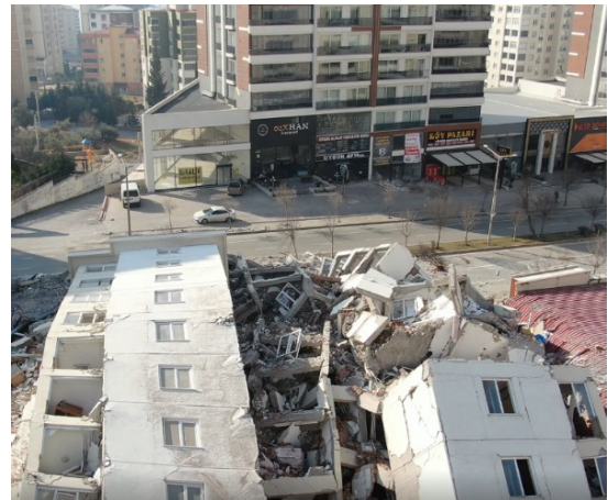
Figure 20. Kahraman Maraş onikişubat haydar bey mah. The building collapsed due to column cutting.
