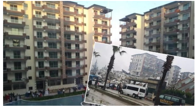
Figure 19. A nine-storey building in Antakya
