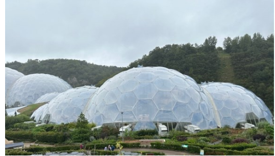
Figure 8. The space-grade structure in Eden Project, Cornwall UK.
