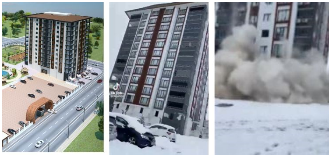
Figure 3. The building built in 2022 in Malatya's Bostanbaşı Neighborhood.
