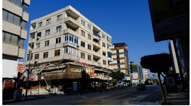
Figure 4. A soft floor incident that occurred in the city center of Iskenderun
