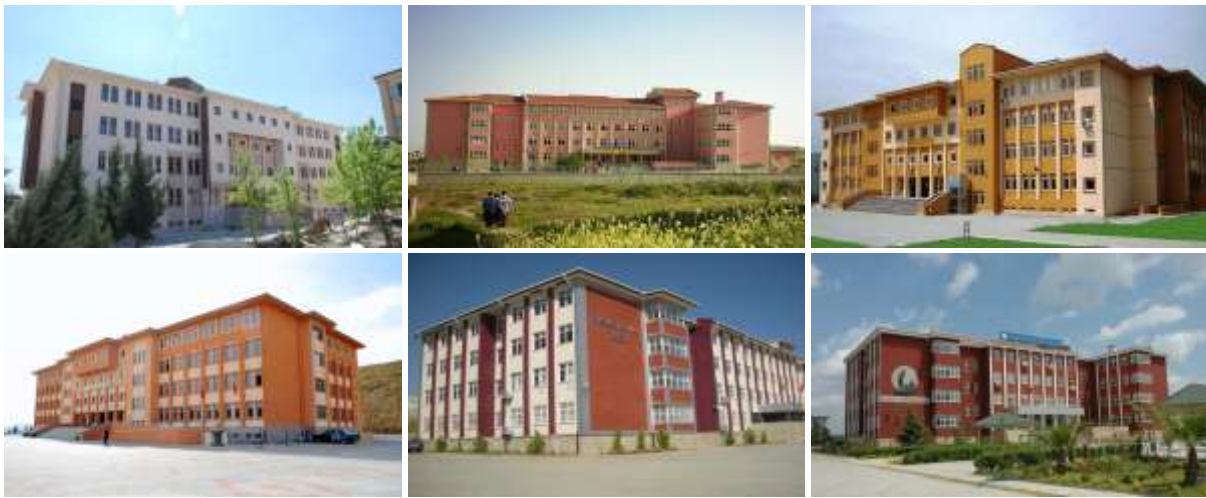
Figure 2. MEB.2000-type upper secondary schools a) MEB.2000.05 with 12-classrooms b) MEB.2000.07 with 16-classrooms c) MEB.2000.08 with 16-classrooms d) MEB.2000.09 16-classrooms e) MEB.2000.11 with 24-classrooms f) MEB.2000.12 with 24-classrooms (Sourced from personal records of the MEB officials).
