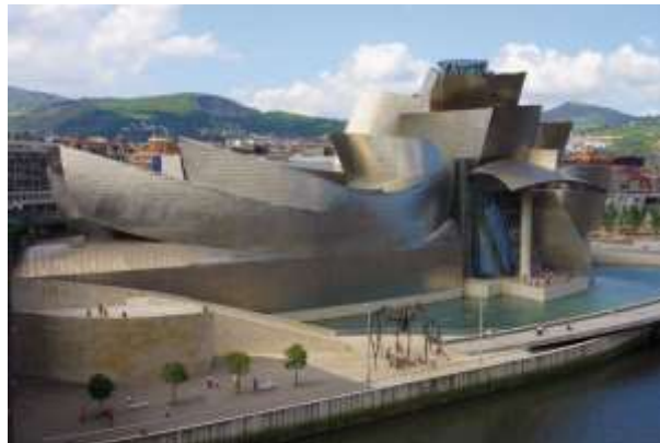
Figure 5. Guggenheim Museum, Frank Gehry, Bilbao, 1997 ( https://www.britannica.com/topic/Guggenheim-Museum-Bilbao )
