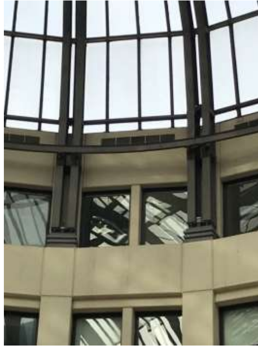
Figure 10. The steel arches of the vault (Nałçacıođlu, 2022)
