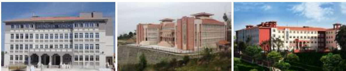
Figure 3. MEB.2004-type primary schools a) MEB.2004.40 with 8-classrooms b) MEB.2004.49 with 24 classrooms c) MEB.2004.50R with 32-classrooms (Sourced from personal records of the MEB officials).
