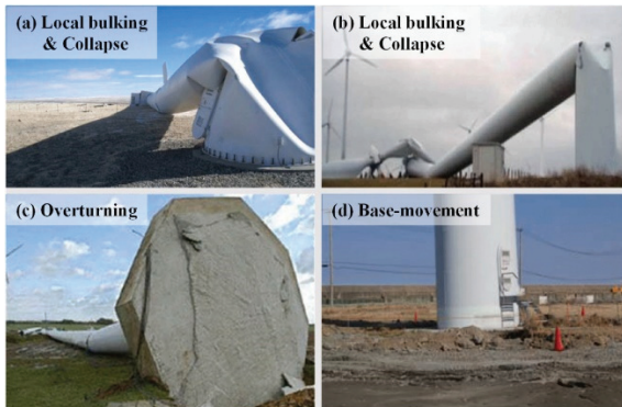
Figure 2 - Possible damage of WPP due to earthquake [16]
