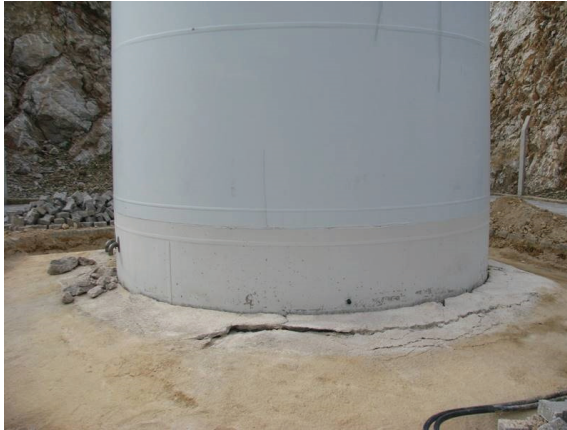
Figure 1 - Damage at the connection of the tower and the foundation of a WPP
