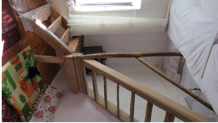
Figure 16. Wooden Stairs in a Traditional Arapgir House.
