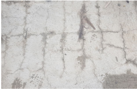
Fig. 7. Plastic settlement cracks
