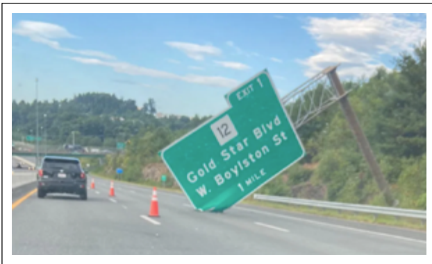
Figure 1. Collapsed sign support.
