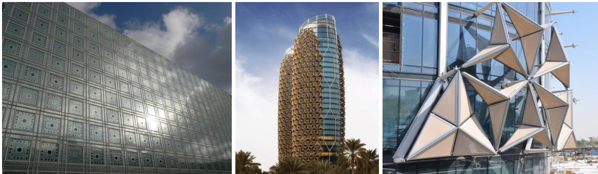
Figure 2. Some pictures of responsive façades: a) Arab World Institute, Paris (FR) [35], b) Al Bahar Towers, Abu Dhabi (AE) [36]. and Al Bahar Towers façade [37].
