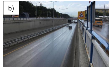
b. Side Wall Visibility -2 (Gürbüz, 2021)
