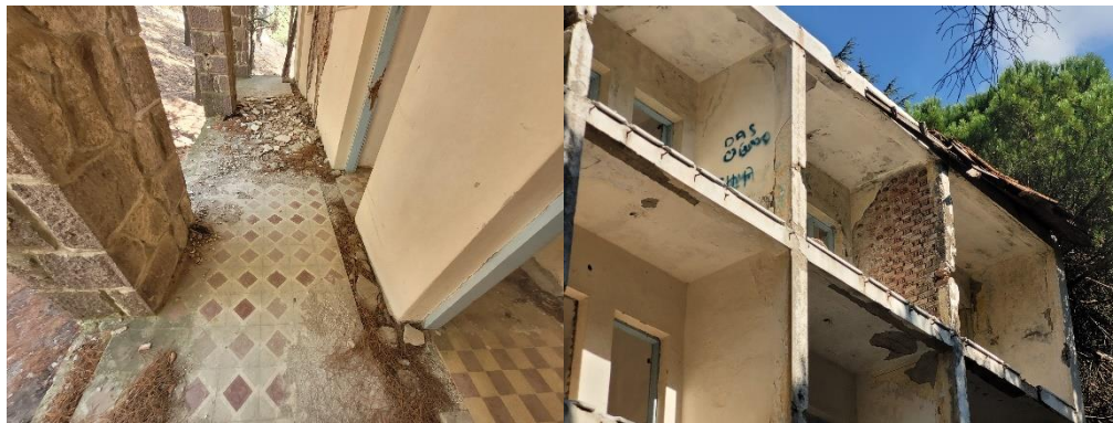
Figure 4. Details from the decaying block-type sanatorium structure that inspired students. Left: Period-style cement tiles in the circulation corridor on the northern side. Right: Brick masonry revealed by a decaying balcony wall on the southern façade (Avcı & Özder Çakır, 2023a)
