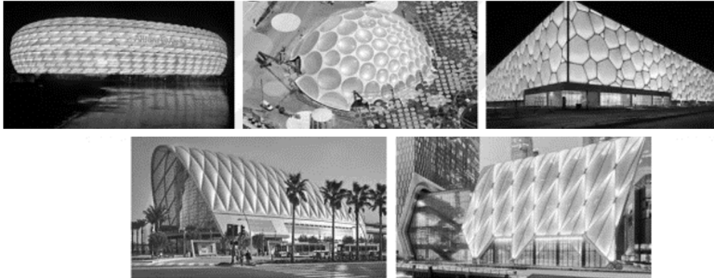
Figure 7. Visuals of the buildings produced with foil material within the scope of the study, 1-Allianz Arena (AGC Chemicals. (n.d.). ETFE film: Allianz Arena. Stylepark.), 2-Thirst Pavilion (Lastra y Zorrilla. (n.d.). Multiple layer covers and facades.), 3-Watercube National Swimming Center (Vector Foiltec. (n.d.). National Aquatics Center), 4-Anaheim Regional Transportation Center (Linden, C. J. ARTICs ETFE pillow assembly ), 5-The SHED (World-Architects. (2021). A movable enclosure of air and plastic.)
