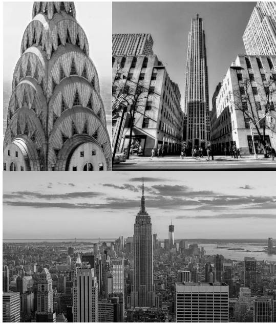
Figure 1. a. Chrysler Building, New York, USA (right) (Chrysler Building, 2024), b. Empire State Building, New York, USA (left) (Empire State Building, 2024), c. Rockefeller Building, New York, USA (bottom) (New York, Rockefeller Center, 2024)
