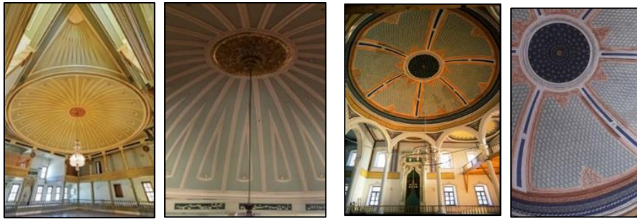
Figure 14. The division of the wooden dome into geometric slices starting from the centre towards the rim in Yenikapı and Gelibolu Semâhanes [7]
