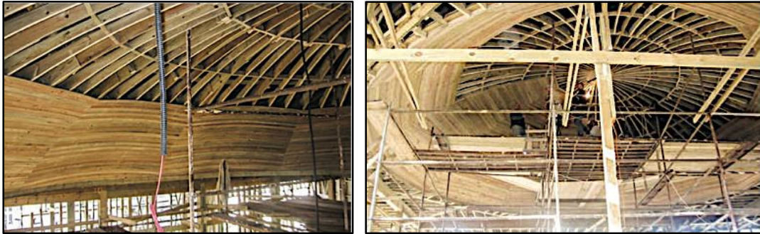
Figure 12. The wooden dome restoration of Yenikapı Semâhane [21]
