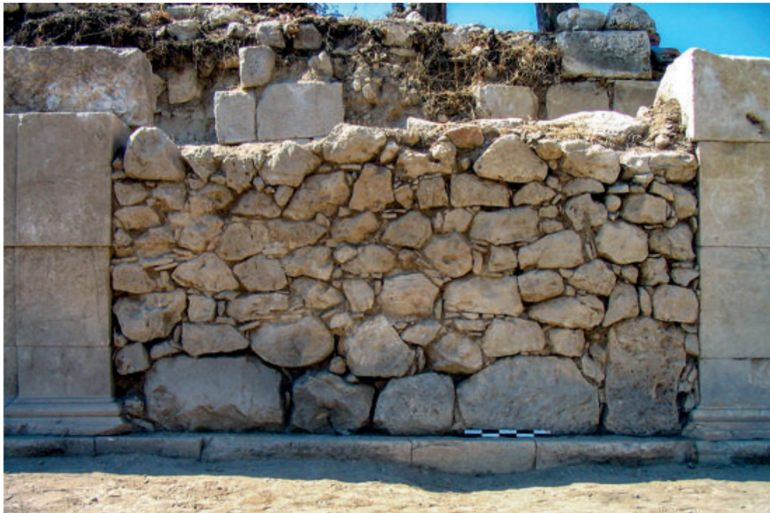
FIG. 31 Eastern entrance of the western stoa of agora, walled-up during the construction of the propylon (© Patara Excavations).
