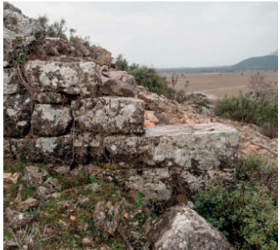
FIG. 14 Ören Tepe. Pseudo-isodomic masonry on approach to south tower. View from west.
