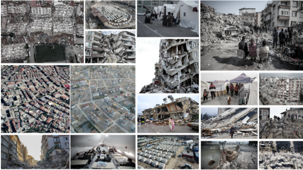
Figure 2. A Visual Study on the Dispositions in Hatay (prepared by authors). From left to right and top to bottom: The destroyed urban pattern, the destroyed buildings, huge voids on the urban ground after the earthquakes, the distorted buildings, the random building stacks, the damaged roads and infrastructures, the disposed urban life, living in the tents and open areas as stadiums, the children studying in the tents as their classrooms.
