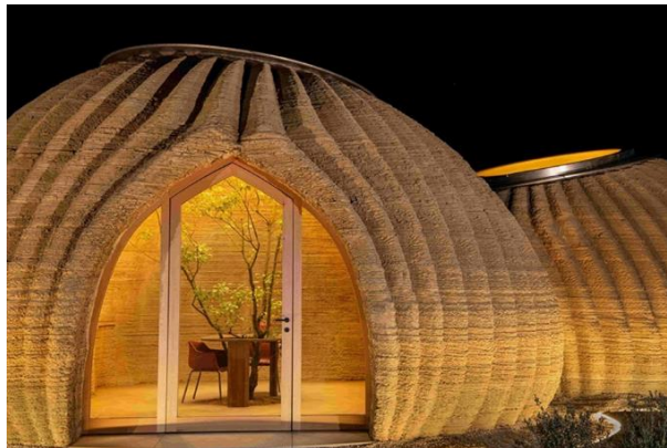
Figure 13. Images of building (Url-8).
