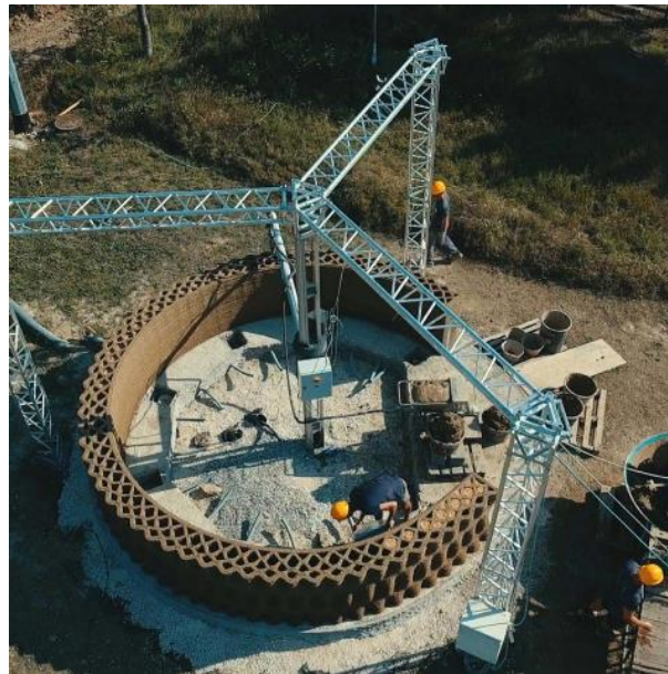
Figure 11. Images of the building (Chiusoli, 2018).
