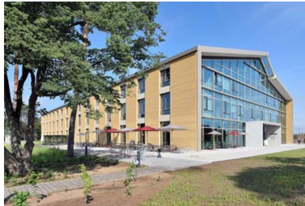
Figure 8. Image of the building (Url-4).
