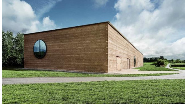
Figure 9. Image of the building (Url-6).
