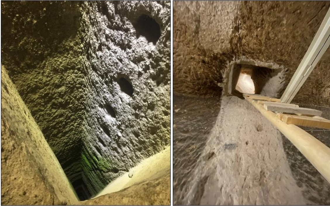
Photograph 4: Ventilation chimneys, Kaymalı underground city (left) and Tatların underground city (right)
