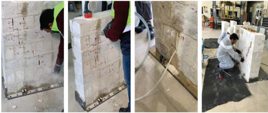
Fig. 4 - The grout injection process [37].
