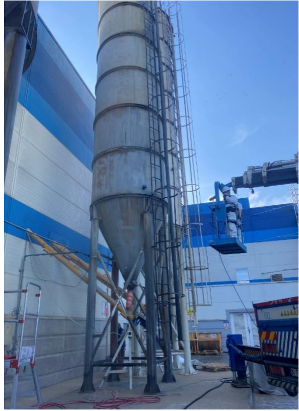
Figure 8. After washing with chemical solution and wiping the silos with a car brush
