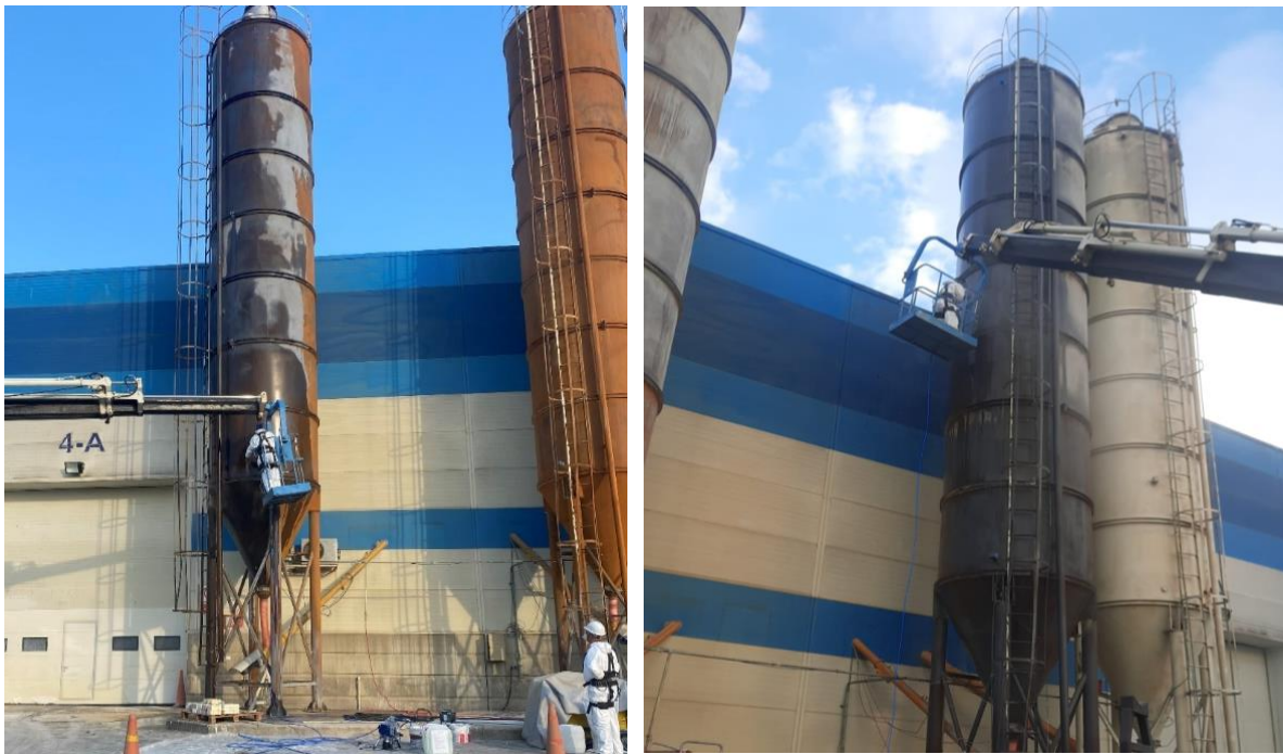
Figure 6. Washing process with chemical solution
