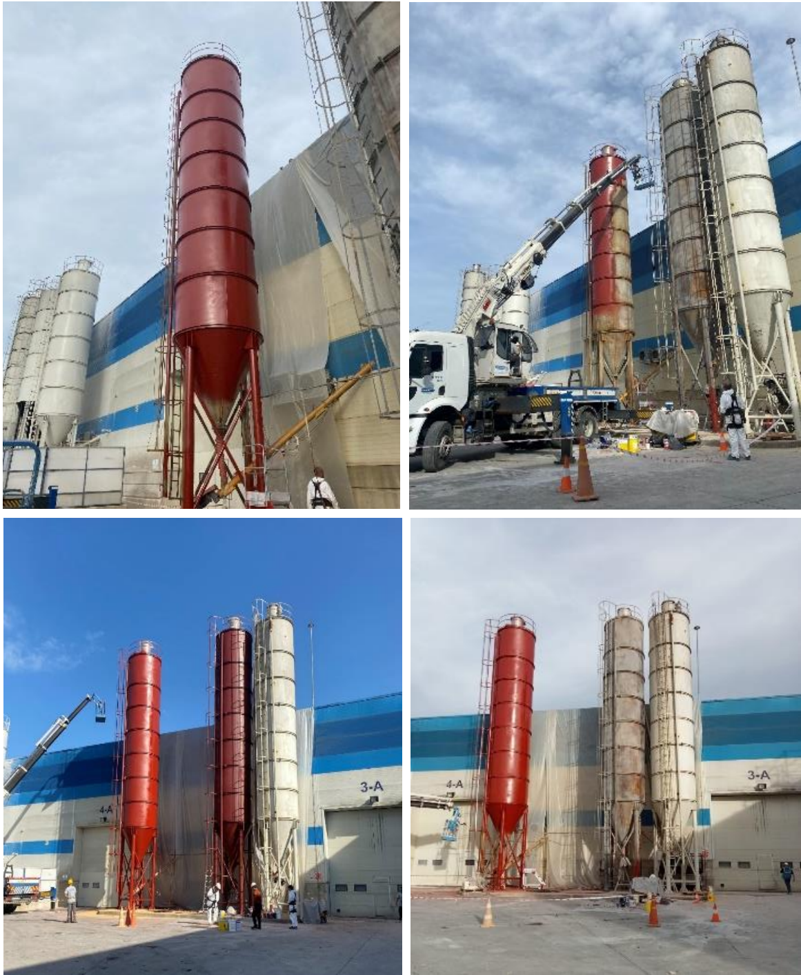
Figure 9. First coat primer application
