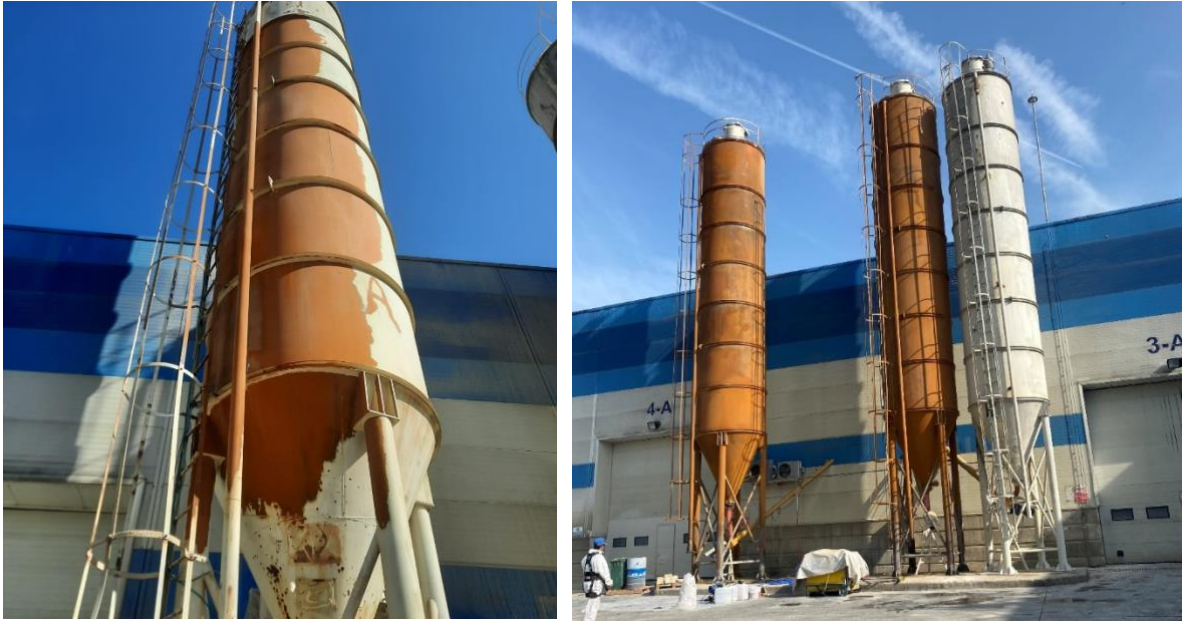
Figure 5. General view of silos after wet blasting
