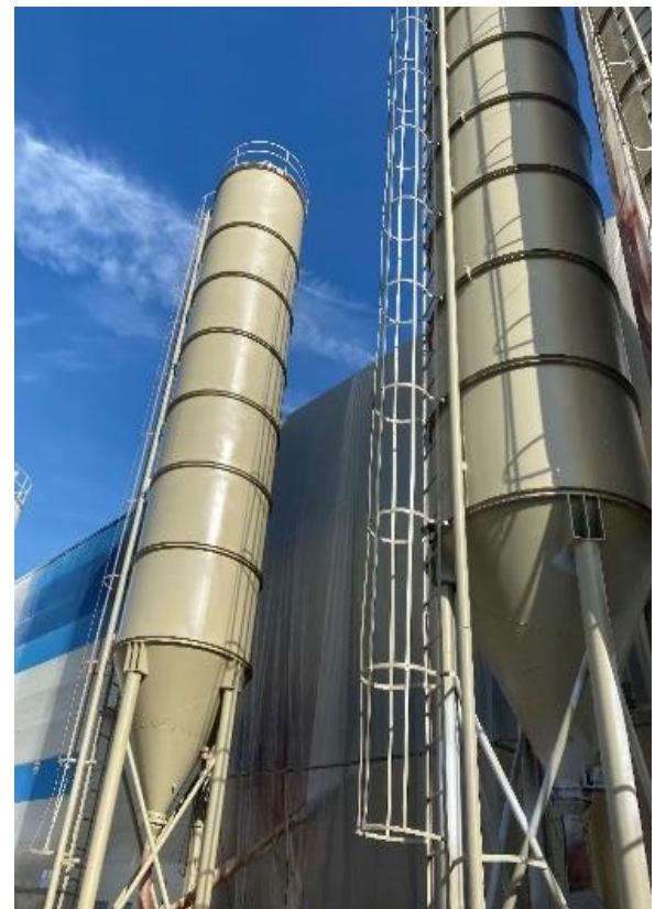
Figure 11. Second coat primer paint application of silos
