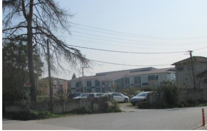
Figure 1. Jet grout soil improvement study area
