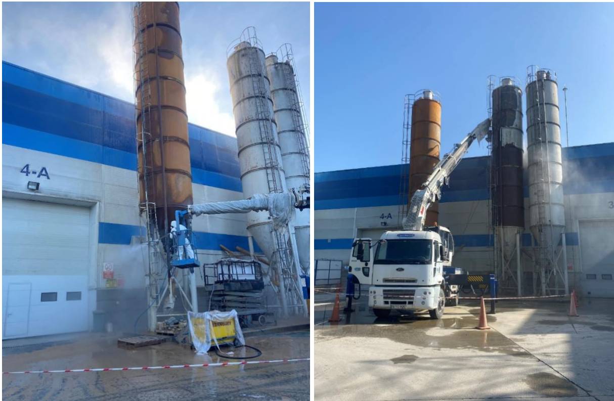
Figure 4. Wet blasting process
