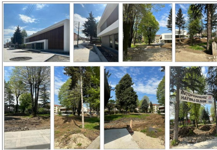
Figure 8. Views of the library and its surroundings located in the Uzun Mustafa neighborhood in the workplace in Düzce
