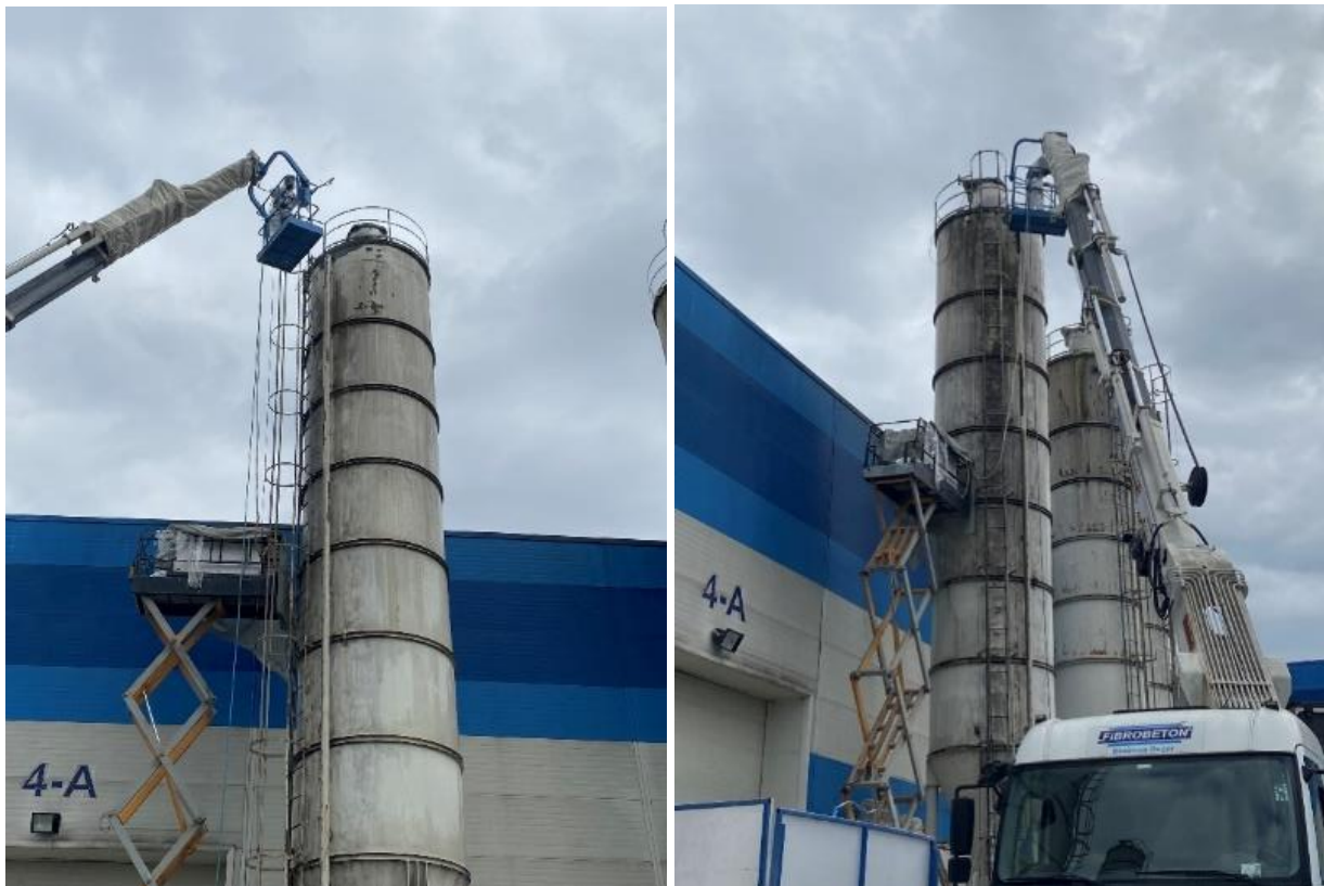
Figure 2. First state of silos
