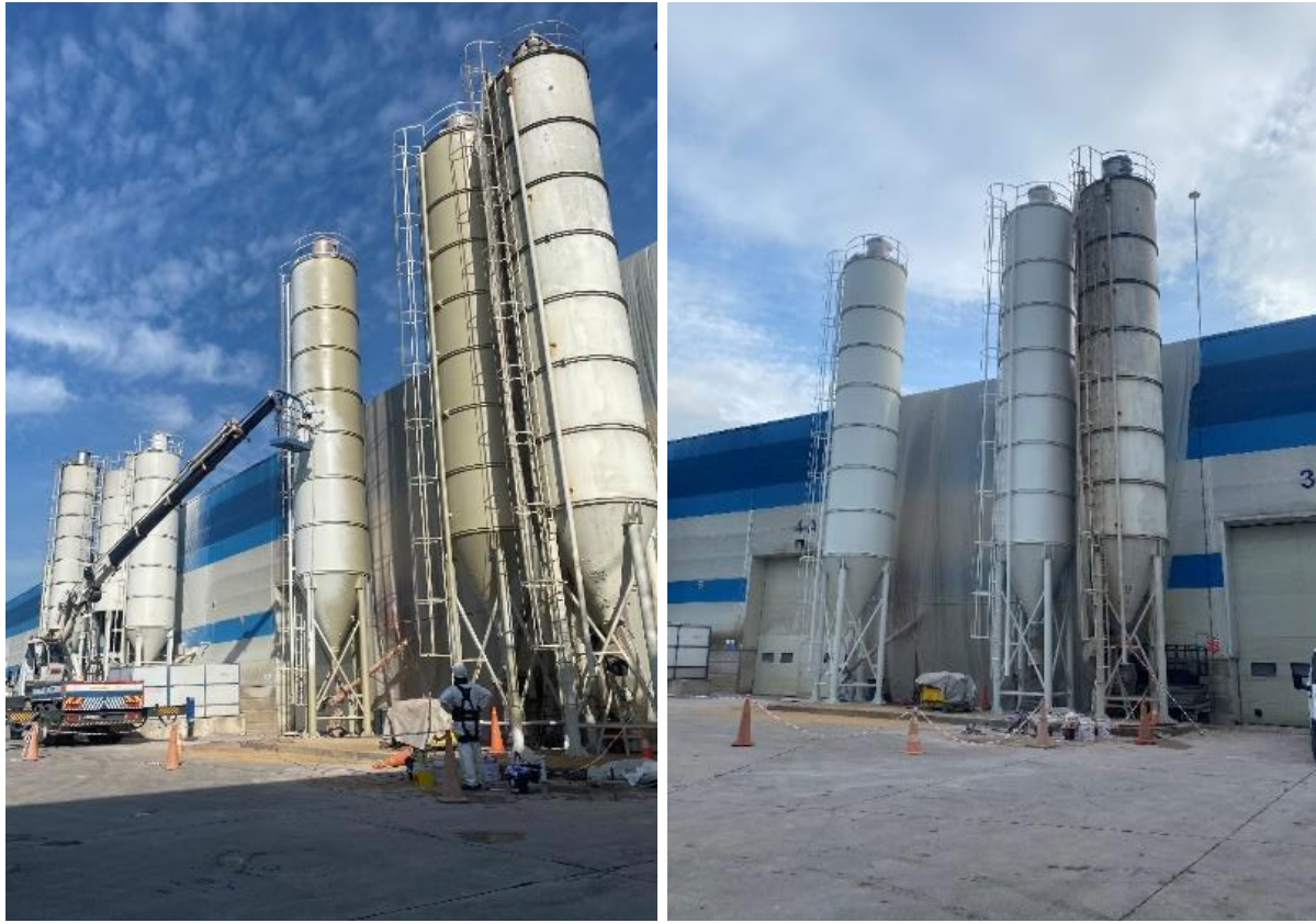
Figure 12. Topcoat paint application of silos
