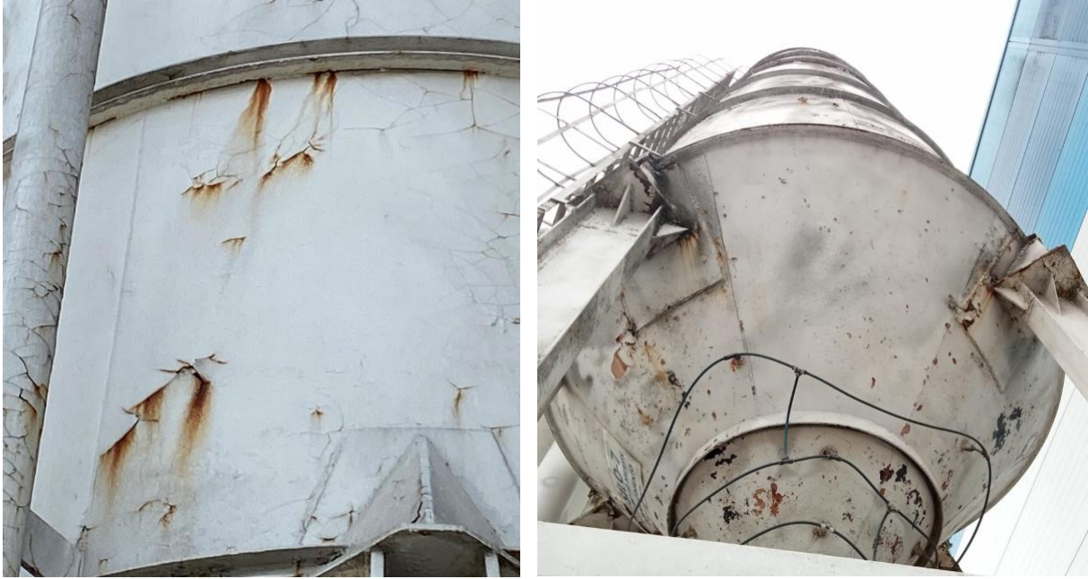
Figure 3. Condition of silos before painting
