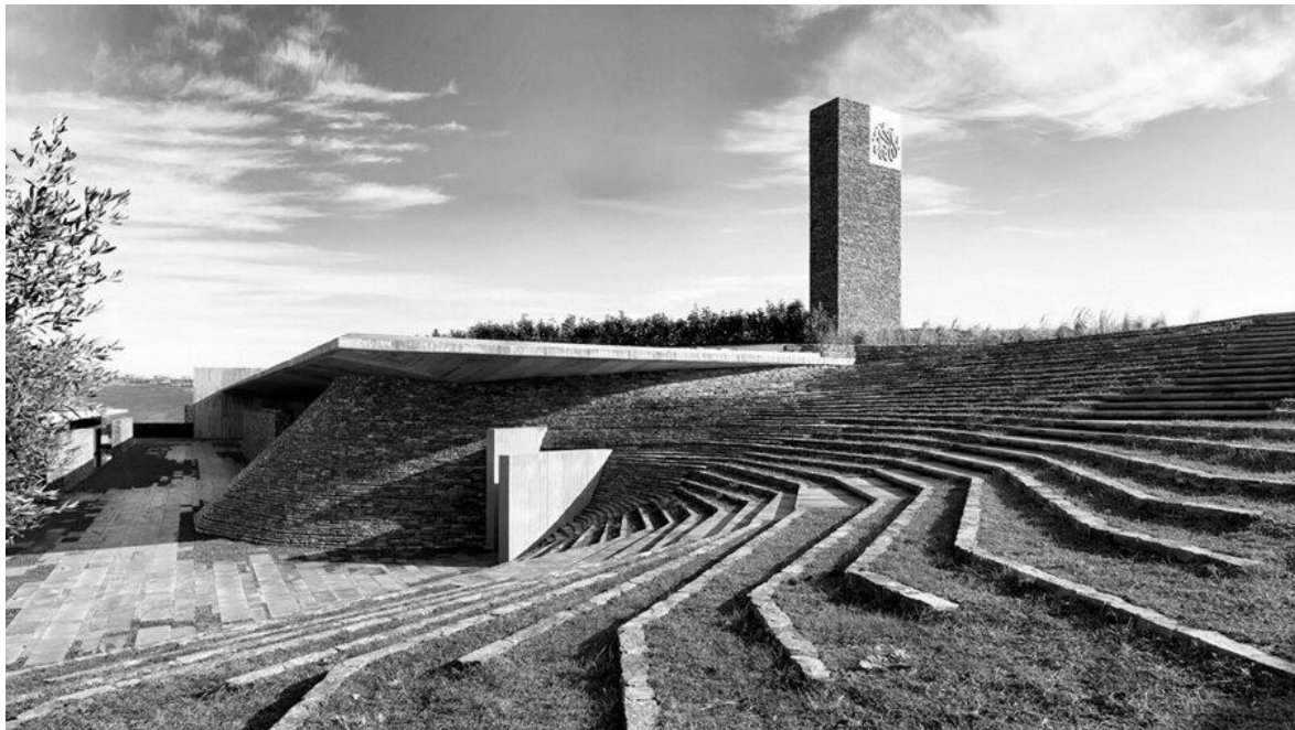
Figure 10. Sancaklar Mosque Stairs (Duman, 2021).
