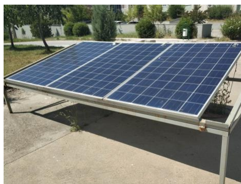
Figure 1. Photovoltaic System Installation.
