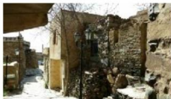
Cement mortar cover the stones
