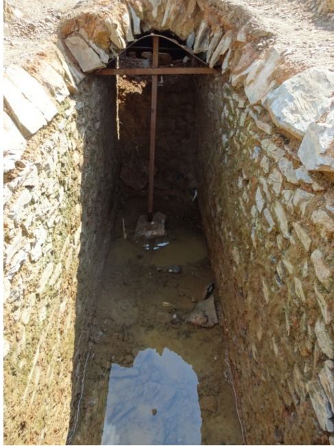
Figure 5: Vault from the original phase of the aqueduct channel.
