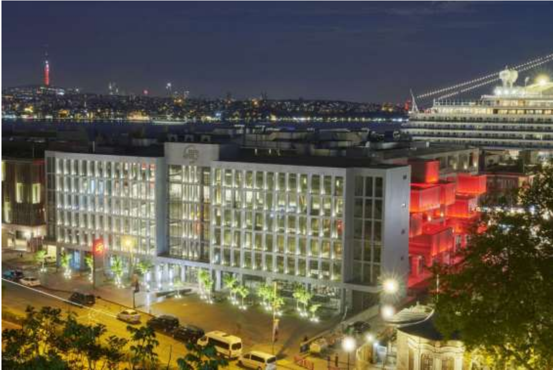
Figure 2. IMPS street side view (Pintos, 2022) Photo by Thomas Mayer.
