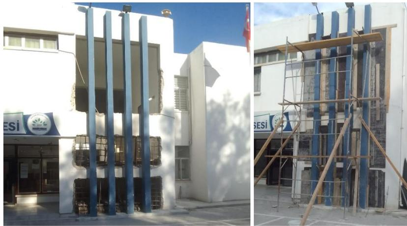
**Figure 12.** Shear wall added to block A; **a)** wall demolishing, **b)** Concrete pouring
