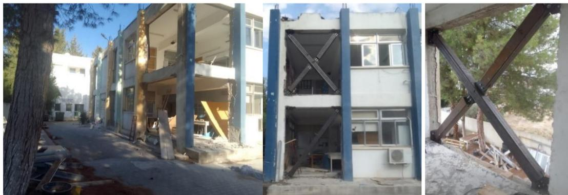
**Figure 13.** X-braced frames added to block C; **a)** wall demolishing, **b)** Braced frame implementation **c)** Tube 200x200x12.5
