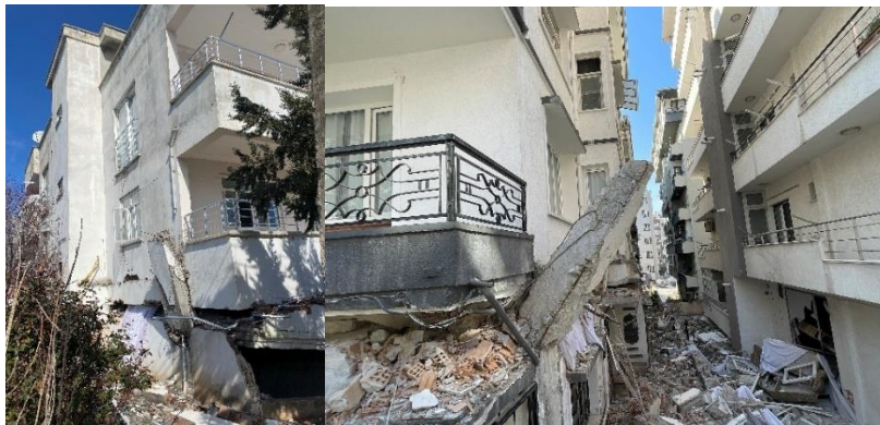
Figure 12. Damage caused by the high vertical earthquake effect.
