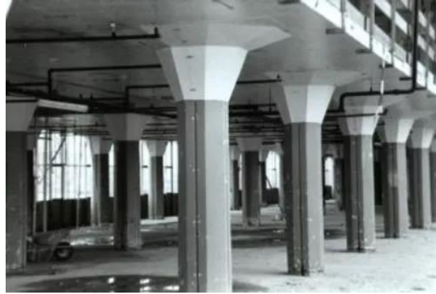
Figure 3. Mushroom Columns, Van Nellefabriek Interior [27]
