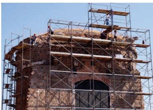
Fig.3. Recent restoration work at Pergamon
