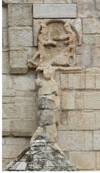
Fig. 5: Malabadi Bridge, Figures.
