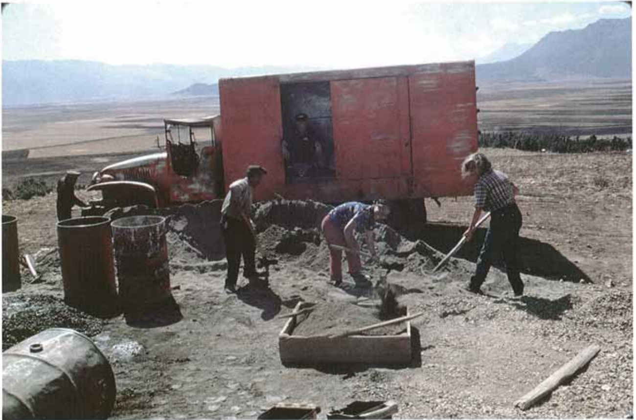
Res. 11: Kızılbet, M. Mellink mixing cement (September 1974).
