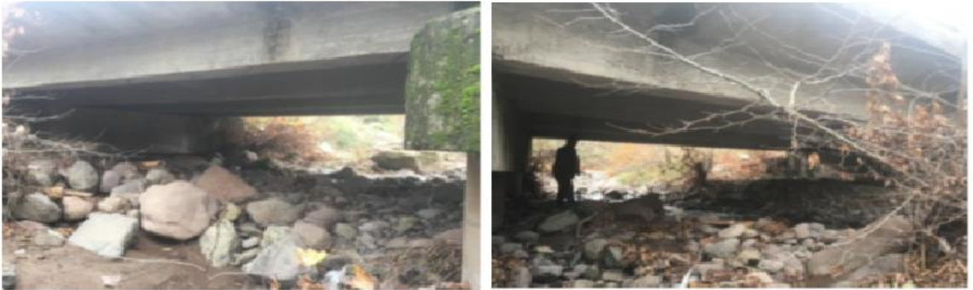
Figure 2. Alandegirmeni Bridge (KM 10+050~10+080) (a) Upstream view of the bridge; (b) Downstream view of the bridge.
