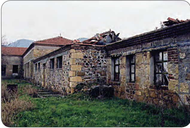
Fotoğraf 6: Ayvacık sahilinde bulunan bir zeytinyağı imalathanesi / An olive oil installation from the shores of Ayvacık (Hacıoğlu 2008)
