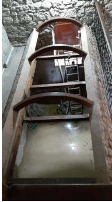
Figure 3. The cistern in the Birdane Mansion (Photo: Author/s archive )
