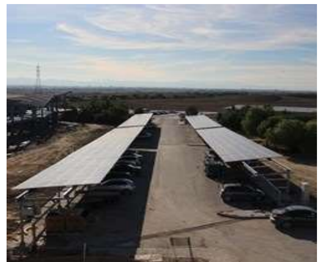
Figure 3. CIU car park spp (solar power plant) installation.
