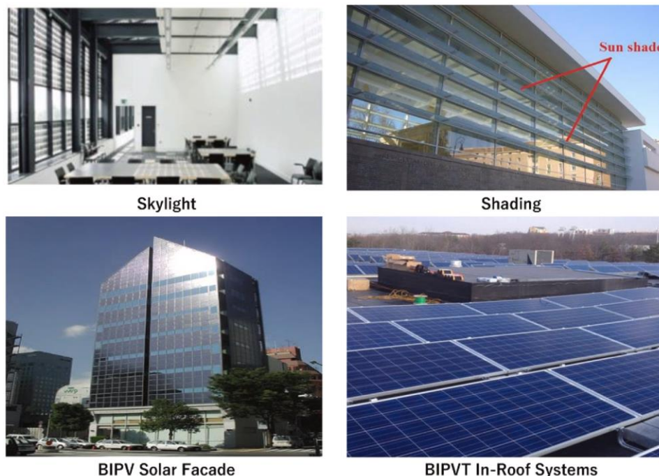
Figure 8. Applications of BIPV/T systems on the roof and façade (Maghrabie et al., 2021).
